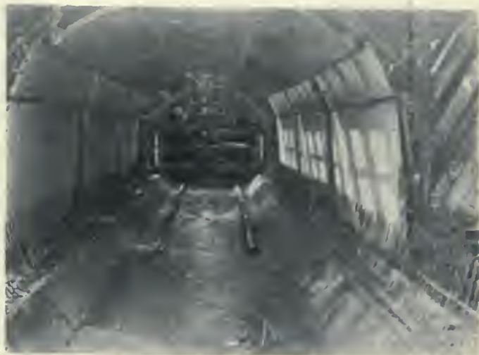
Invert completed and track laid for inner forms. Outer forms being placed—Note reinforcing rods to join the invert to the superstructure.
